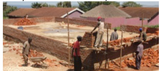
GTS Library project June 24
